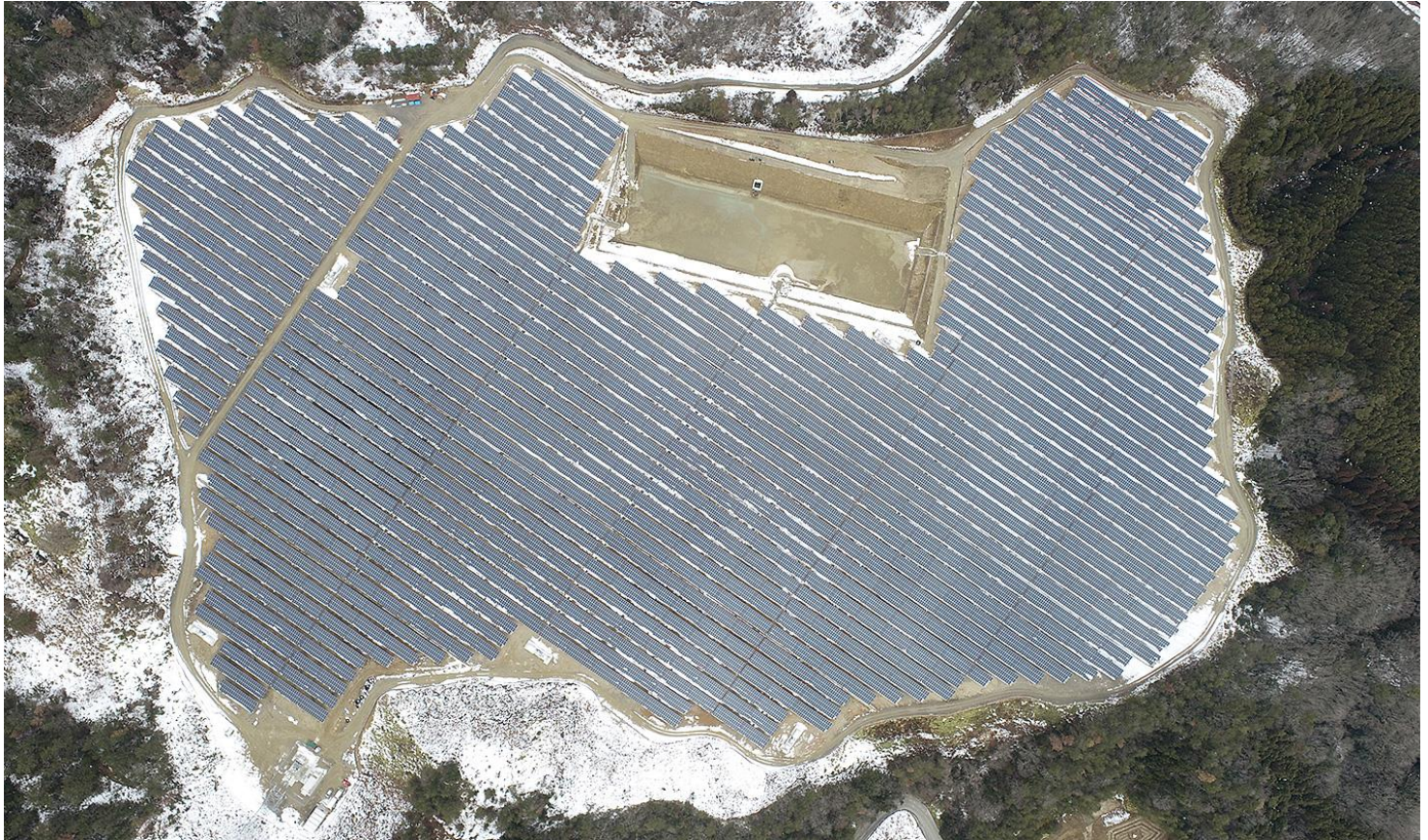
Figure 8. CSIF Hiroshima Suzuhari Power Plant (Hiroshima Prefecture) (17MW)
