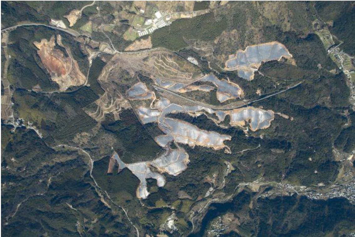
Figure 5: CS Hiji-machi Dai-Ni Power Plant (Oita Prefecture) (53.4 MW)
