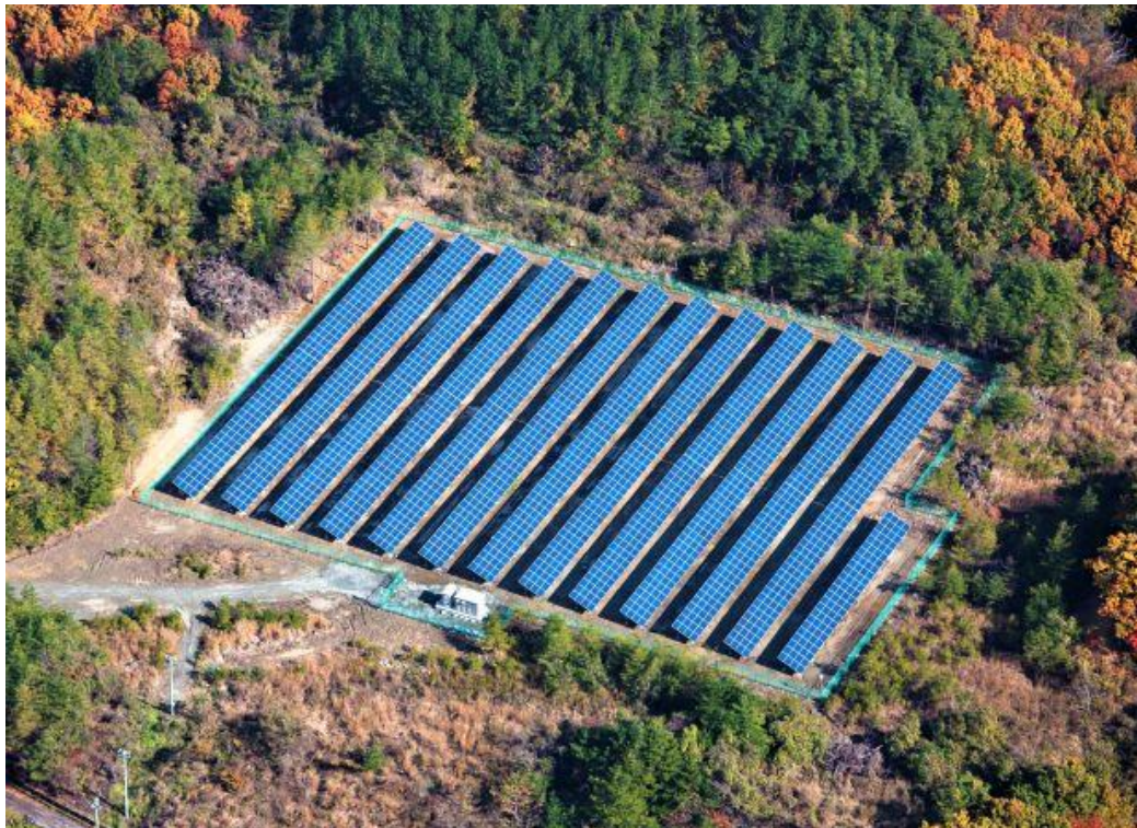
Figure 6: CS Koriyama-shi Power Plant (Fukushima Prefecture) (0.6 MW)
